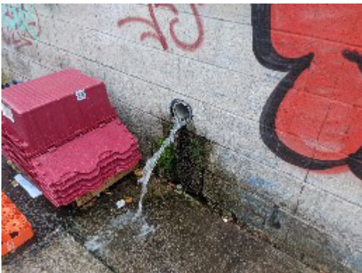
3. Shoppers Drugmart Roof drainage discharges to the parking lot surface
